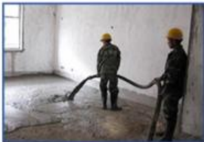
CLC foam concrete floor
